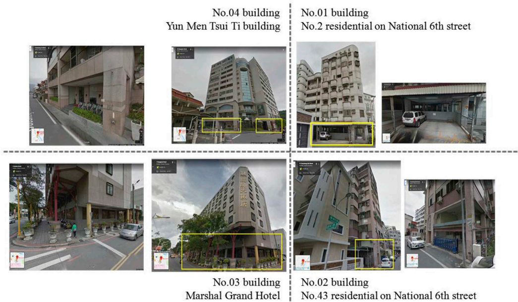
Fig. 14. The bottom-stories layout of four collapsed buildings (from Google Map).
